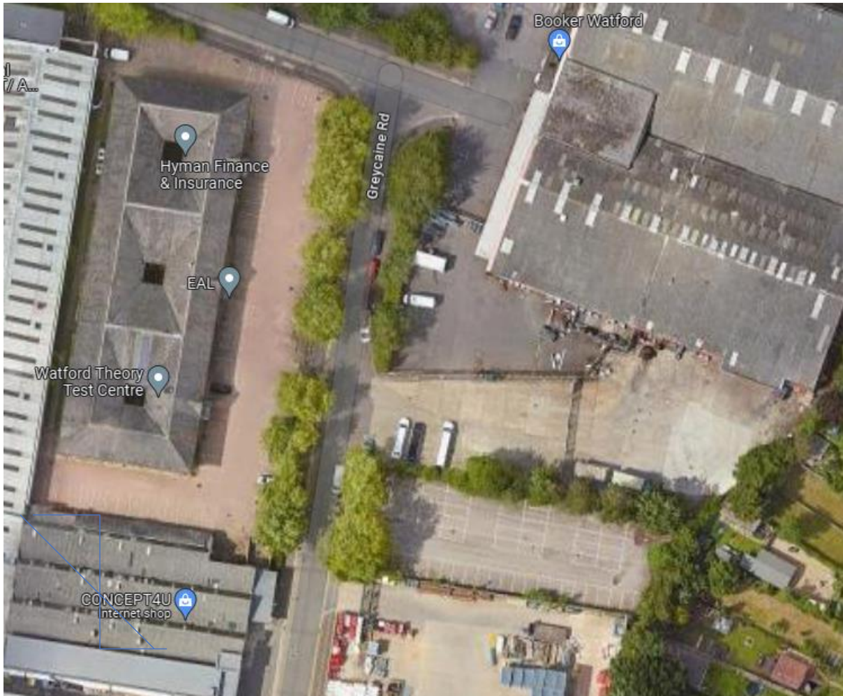
Aerial view of site
